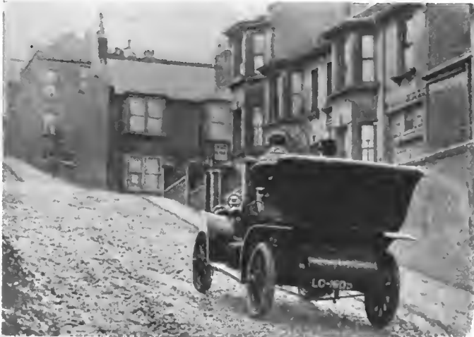
WINTON CLIMBING ONE-IN-FOUR GRADE AT PRESTON, ENG.
